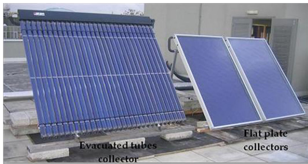
Fig. 1. Evacuated tube and flat plate collectors.
