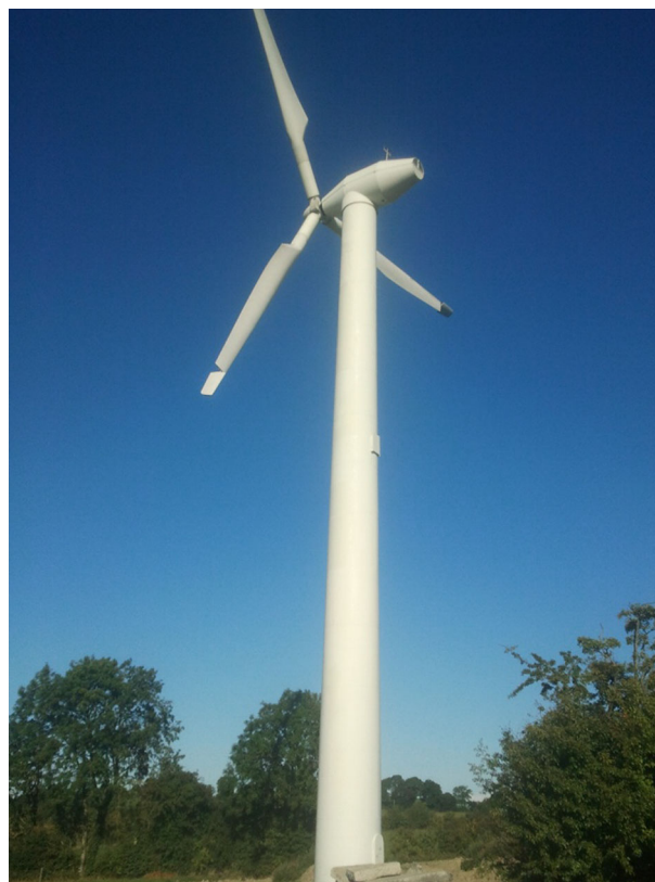
Fig. 1 Picture of 300 kW DFIG on-site turbine
