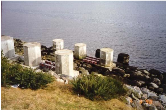
Fig. 14 - Shows the location of the pier stem (right hand side of the picture) near the Dornoch bridge, Scotland
