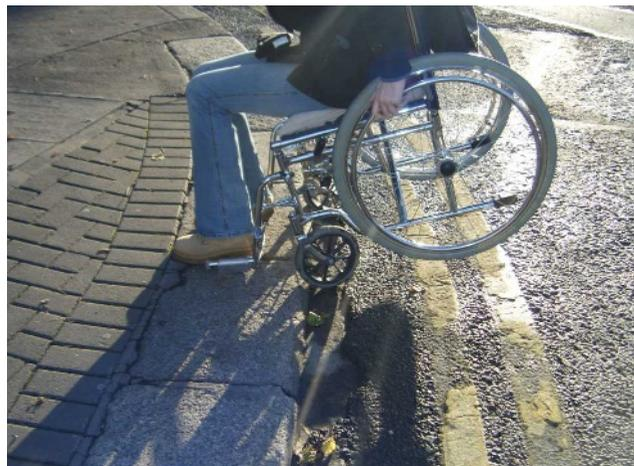
Figure 2. Wheelchair user trying to mount a pavement without a kerb cut
