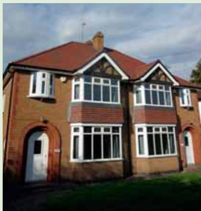
methodology is also interesting. They adapted two adjoining, semi-detached houses to create a matched pair of test houses for full-scale, side-by-side overheating experiments under real weather conditions. Synthetic occupancy was applied with dynamic remote control of actuated windows, motorised curtains, automated internal doors and internal heat gains. The houses were provided with calibrated sensors to measure the internal and external conditions.
