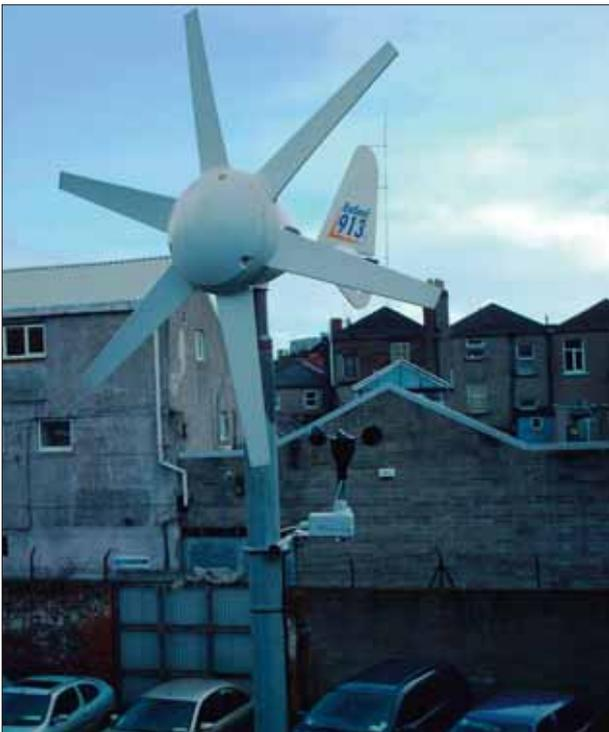
Figure 8: 220W wind charger installed in Church Lane, DIT Kevin St Campus
